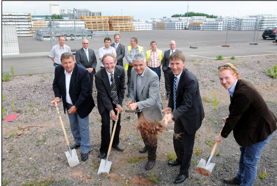
The first cut of the turf marking the official go ahead for profine's new logistics area in Pirmasens on 31 May 2012: From left to right: Wolfgang Hoppe, engineering office Hoppe & Link; Werner Berger, Head of the profine Building Department; Dr Bernhard Matheis, Lord Mayor of the City of Pirmasens; Gerhard Schwager, profine COO; Clemens Walter, Walter Real Estate.
