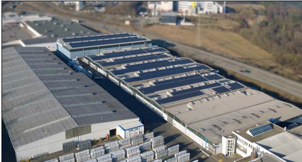
For the EEG-compliant photovoltaic system, a total of 4,583 modules were installed on five roofs at profine GmbH's Pirmasens site.
